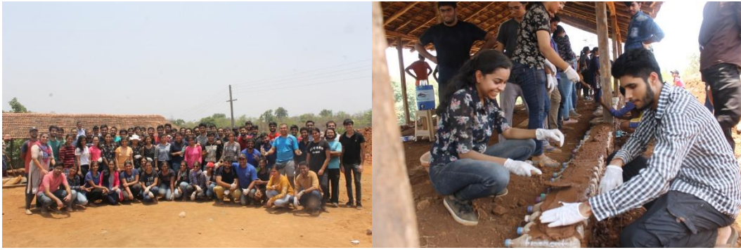
JPMorgan volunteers constructing a wall of the recycled plastic bottle cottage
